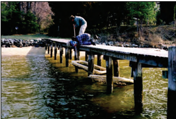
Workers hoist floats onto dock for inspection.
