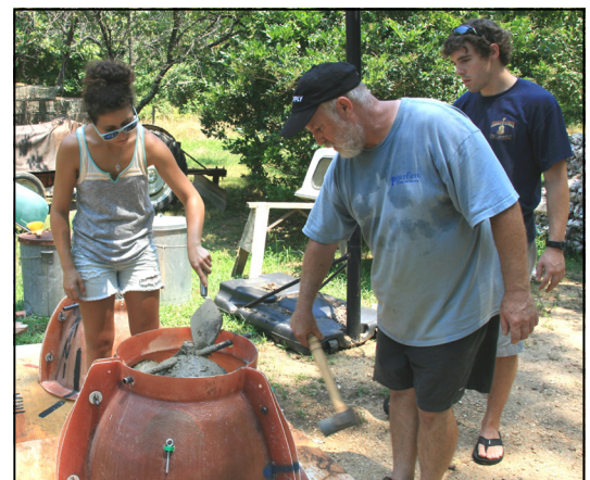
Allison Rugila, Bob Lewis, and David Wood build a reef ball by adding cement to the orange mold.
